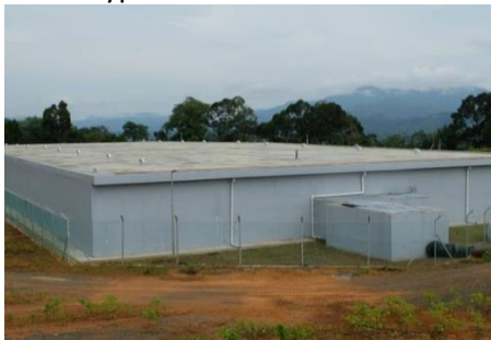
Other Types of Tank
