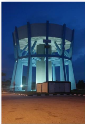
RC Elevated Reservoirs
