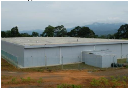
Other Types of Tank
