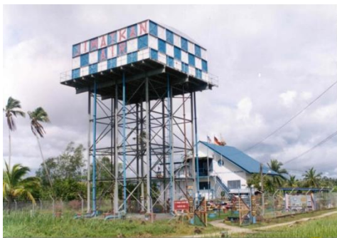
Pressed Steel Tank
